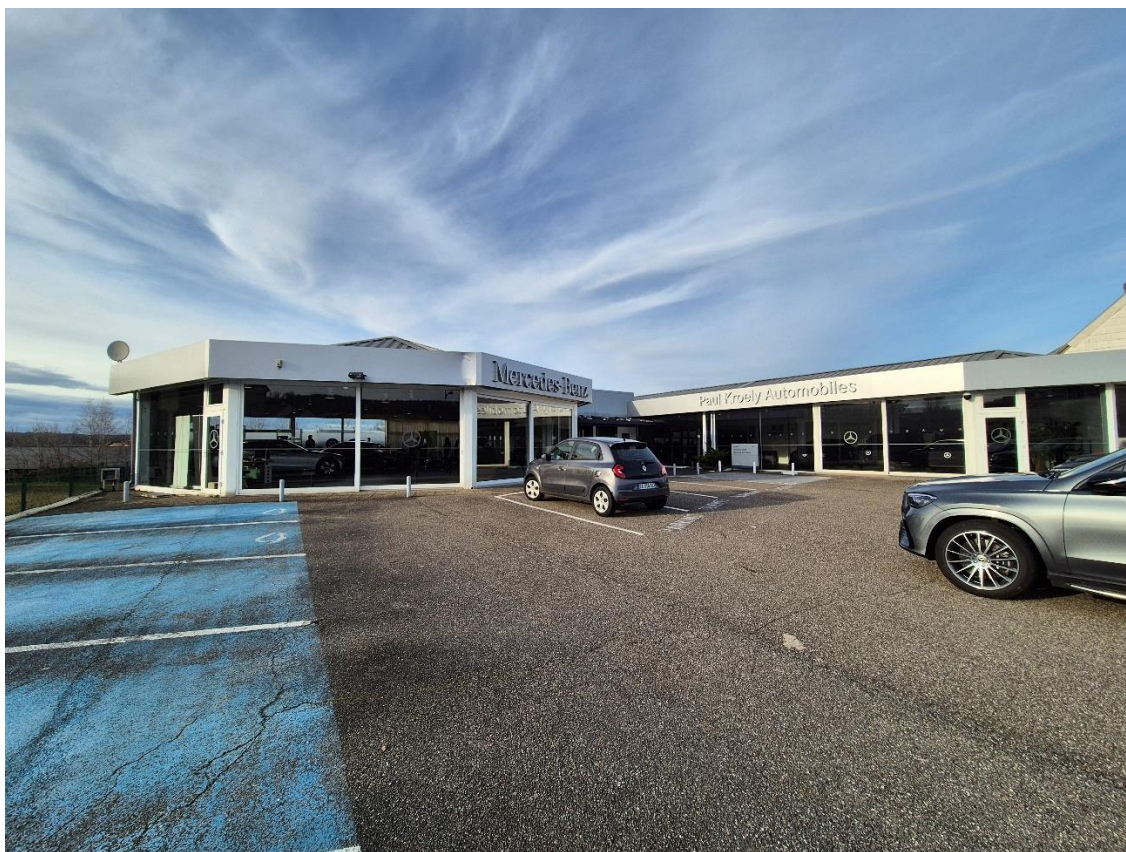
Figure 5: Face SUD-EST / Vitrine commerciale + parking client
