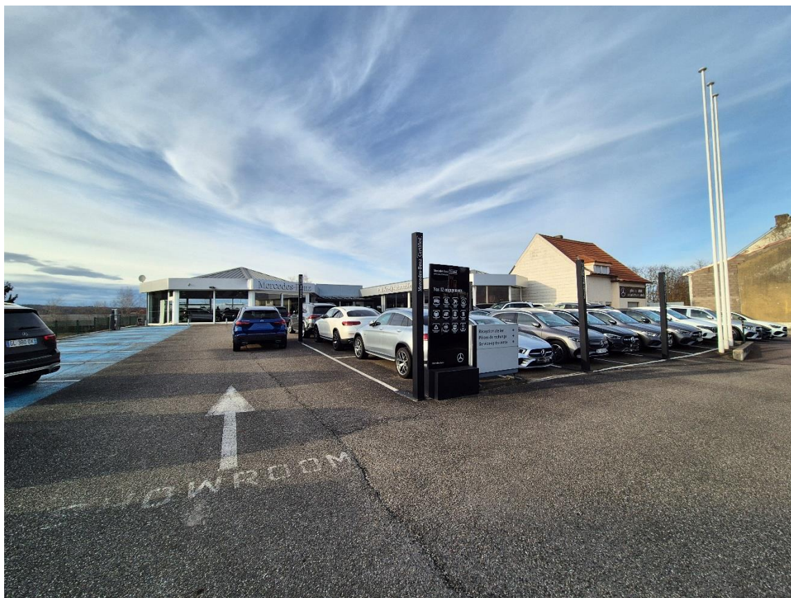
Figure 7: Face SUD-EST / Vitrine commerciale + parking client
